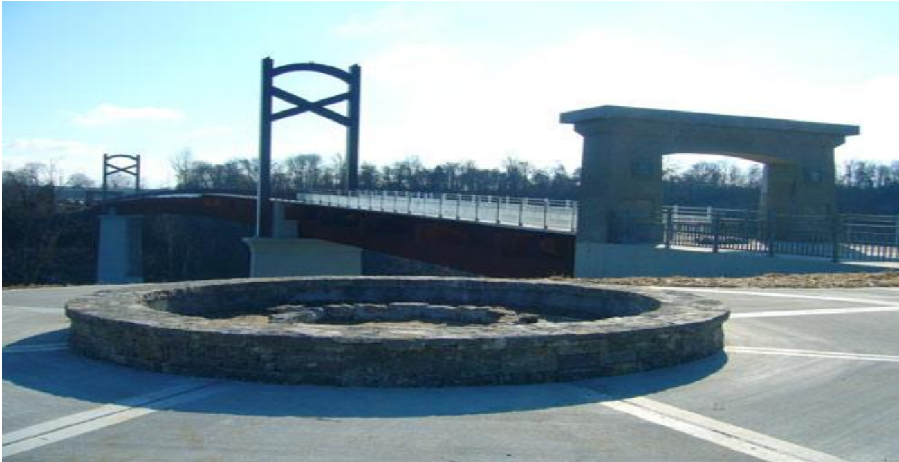
Cumberland River Pedestrian Bridge – Stones River Greenway
