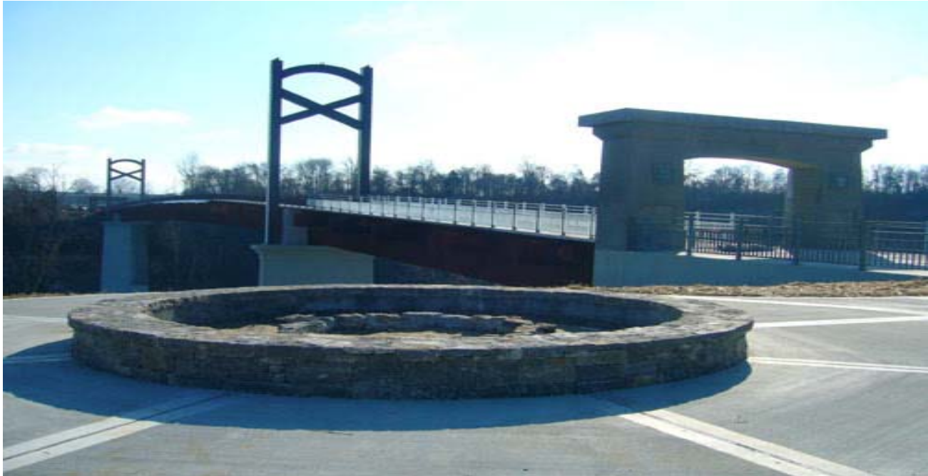
Cumberland River Pedestrian Bridge – Stones River Greenway
