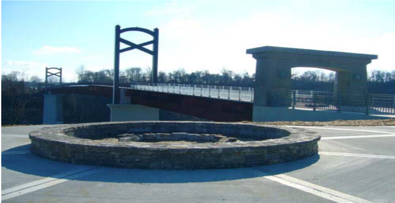
Cumberland River Pedestrian Bridge – Stones River Greenway
