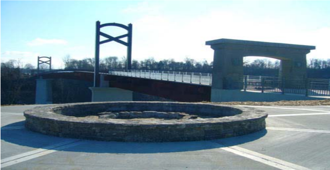
Cumberland River Pedestrian Bridge – Stones River Greenway
