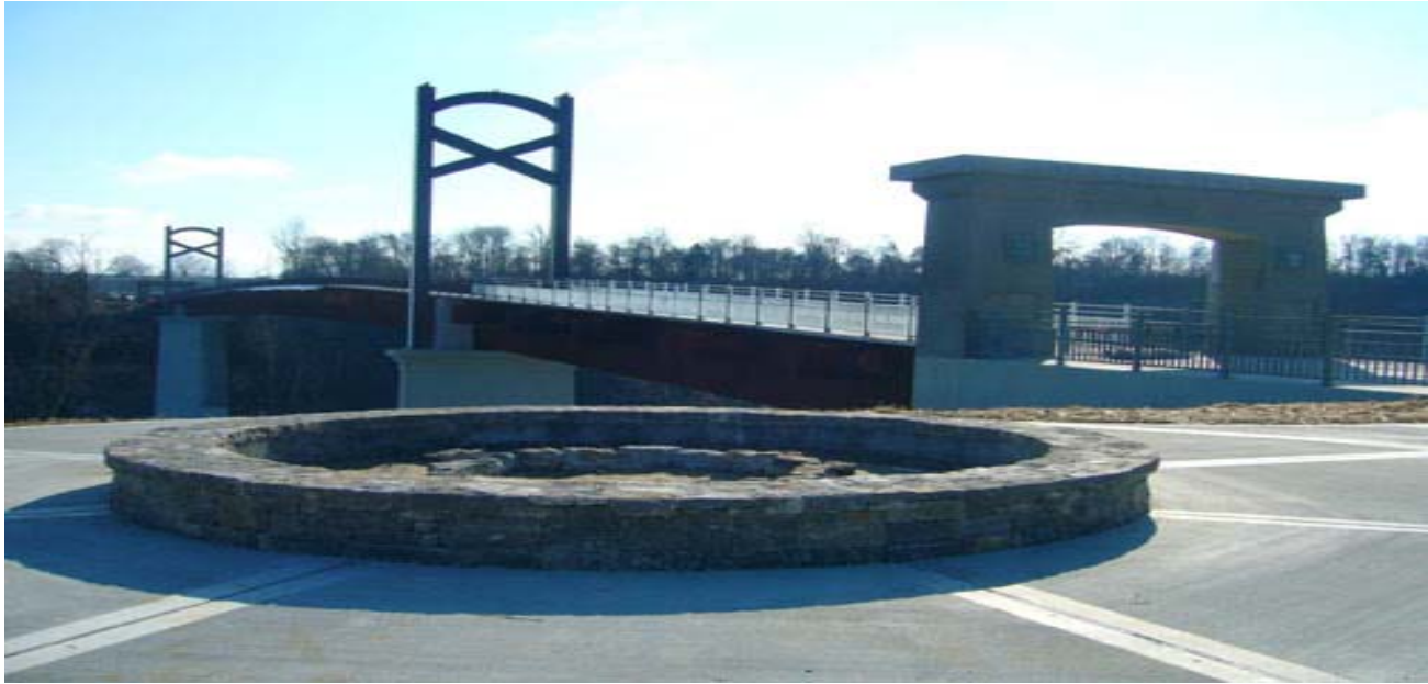
Cumberland River Pedestrian Bridge – Stones River Greenway
