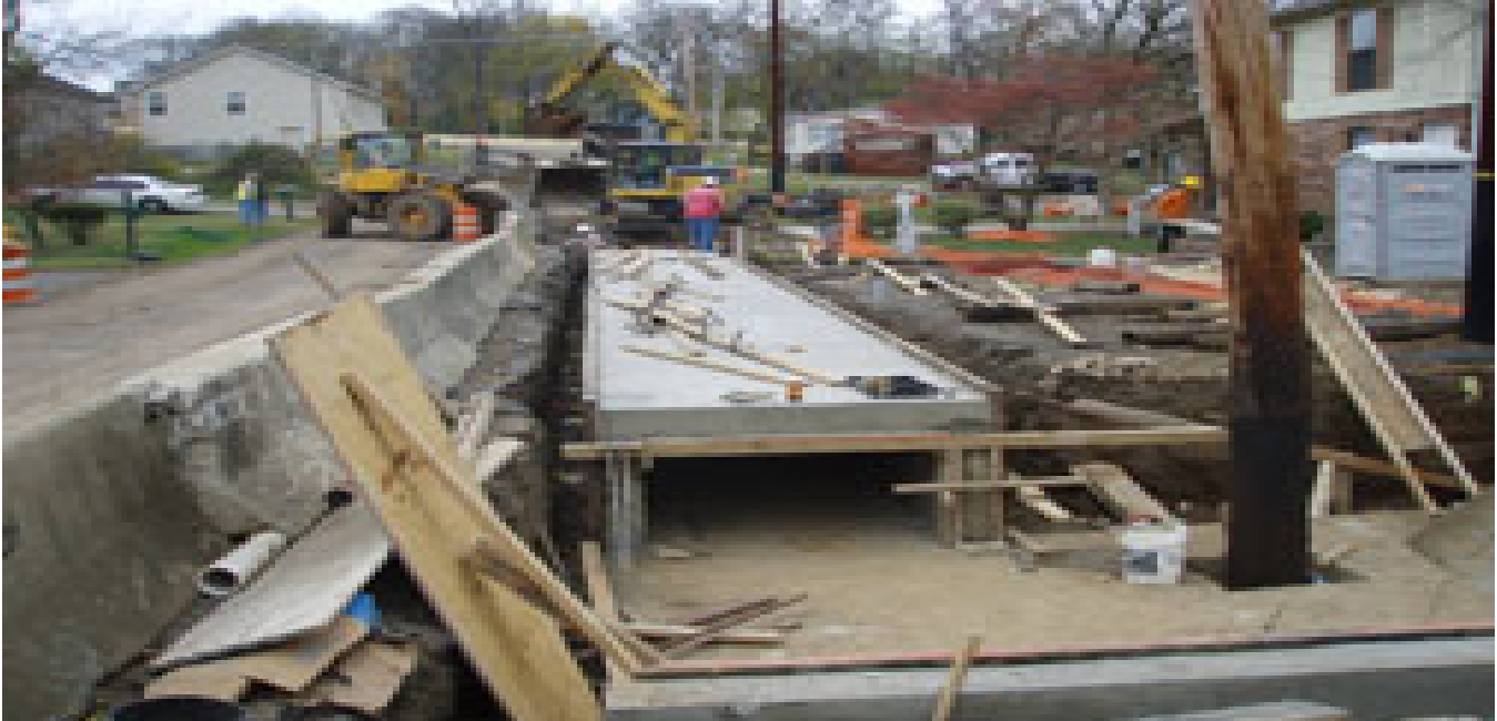
18th Avenue North Stormwater Project
