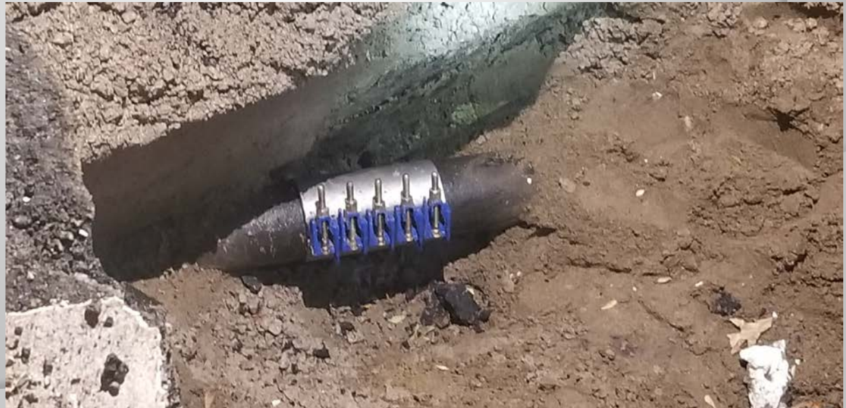
Repair Clamp on 6" CHW at 4 th and Union
