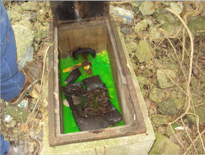
Drain Valve Leak near Nissan Stadium
