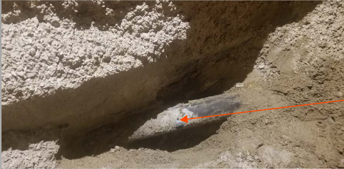
Excavated 6" CHW at 4 th and Union
