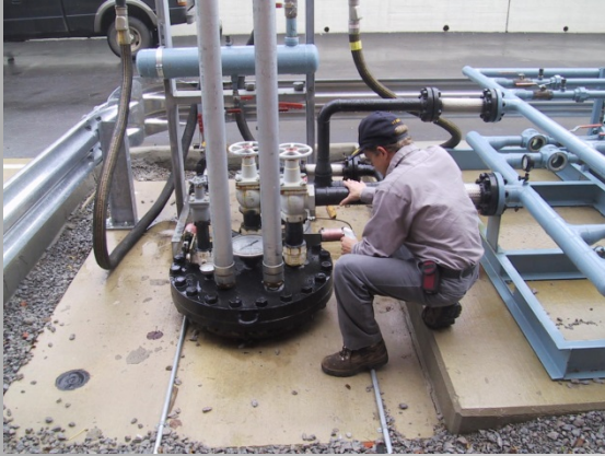
UNDERGROUND STORAGE TANK
