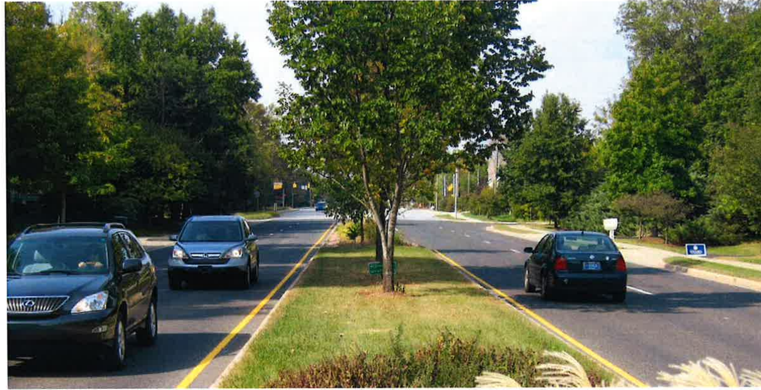
The Parkways in the development will have two travel lanes in both directions, a landscaped median to accommodate turn lanes, planting strips and sidewalks on both sides of the street. The design of the street will accommodate vehicular traffic and provide safe and attractive mobility for cyclists and pedestrians.
