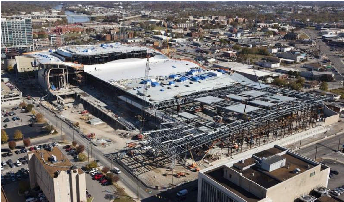
Exhibit B – Aerial View of Construction Progress
