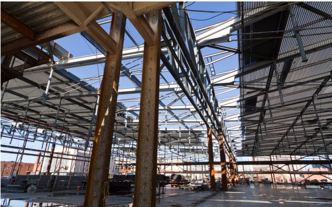
Exhibit C – Roof Installation at the Main Exhibit Hall
